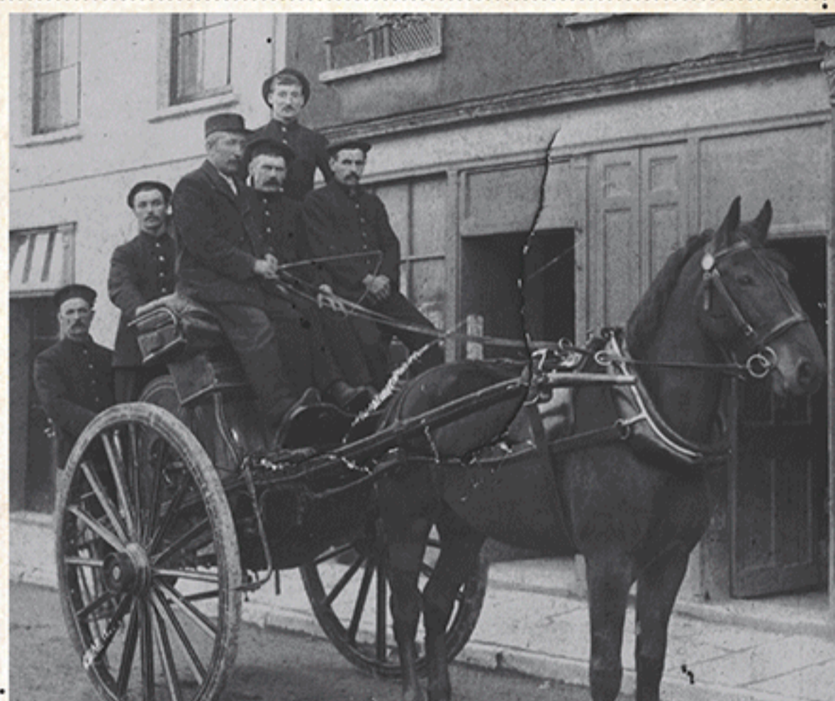
The most common fire appliance at the disposal of the Cork City Fire Brigade in 1920 was one like this, photographed in 1906, with a hose reel underneath the carriage. (Courtesy of Pat Poland)
