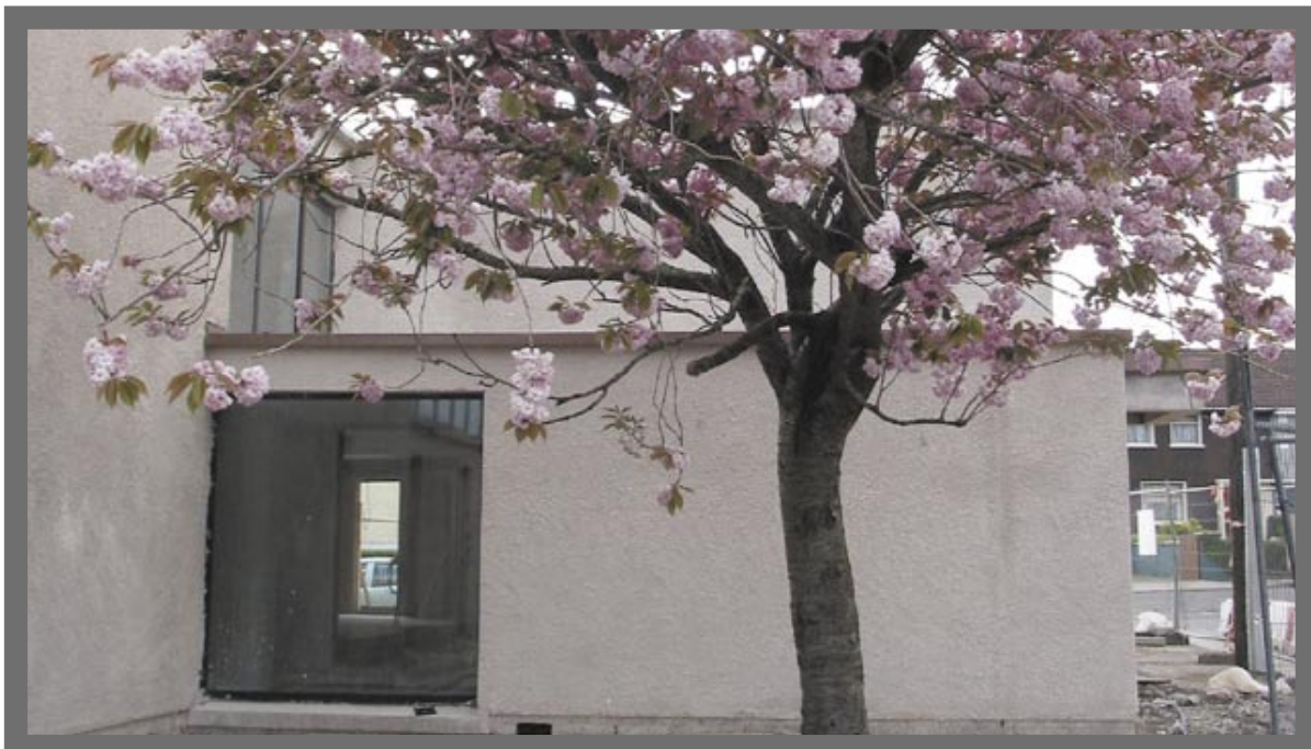
The new Library at Tory Top Road during Construction.
